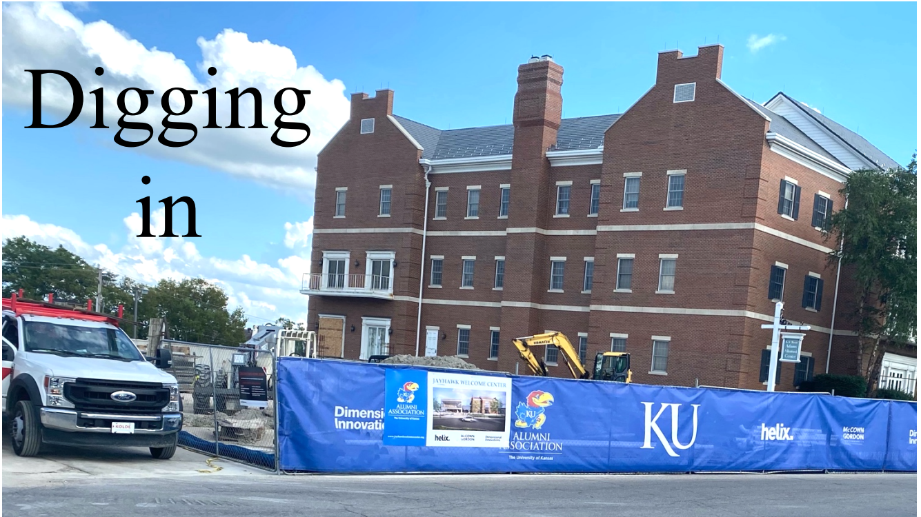
(Above and right) Welcome Center construction site August 2021.
